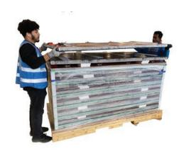
9. Using the protective corner cardboard pieces as support, cut the plastic film at the same height of 2 panels.
