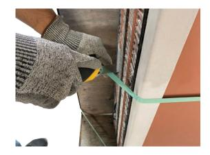
5. Then cut the second strap. Make sure the modules are held by your partner at all times during the cutting to ensure the modules do not fall to the floor.
