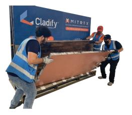
The glass facing of the module can be damaged if it is not placed properly. Make sure that if the panel is facing down, there is not any screw or metallic piece that can damage the surface.
