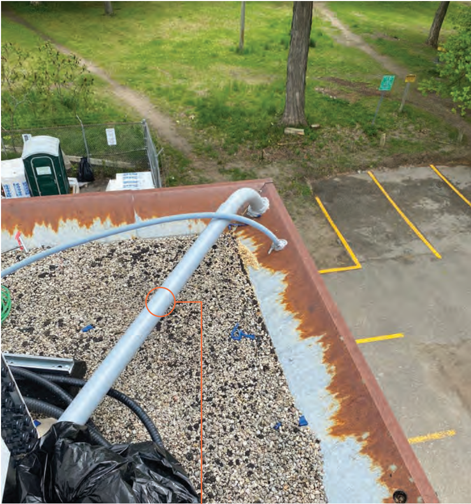
Wiring Set Up To The Building
