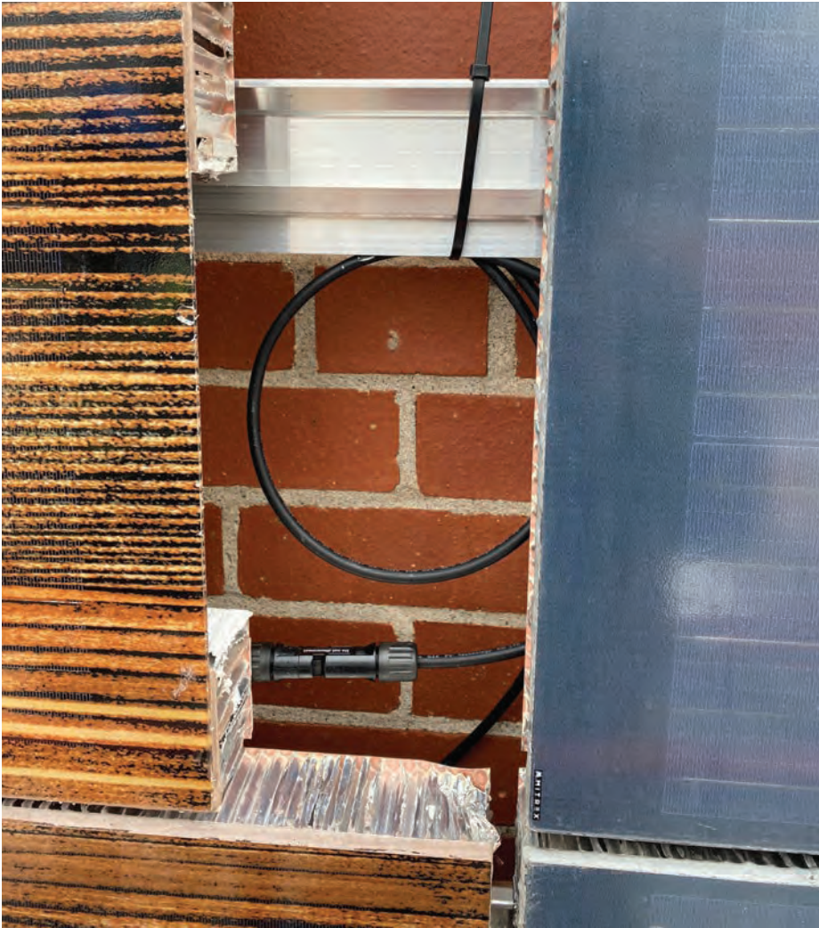
Panel to panel wiring hid behind the panels & run through conduit.
