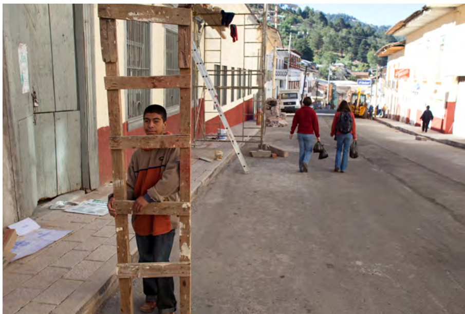
Ann and Christine pass through a construction zone.
