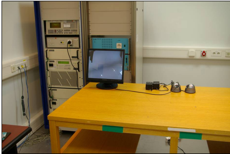
Picture 5. Harmonics & Flicker
